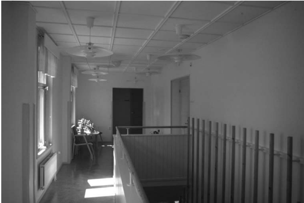
In Alatornio (1786) parsonage, renovation in the 1990's was far too extensive. Almost all the old materials were dumped, apart from the log frame. The interior doesn't differ anymore from the new houses of the 1990's.
