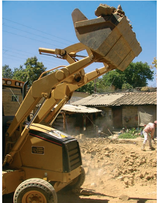
Demolition of an adobe house
