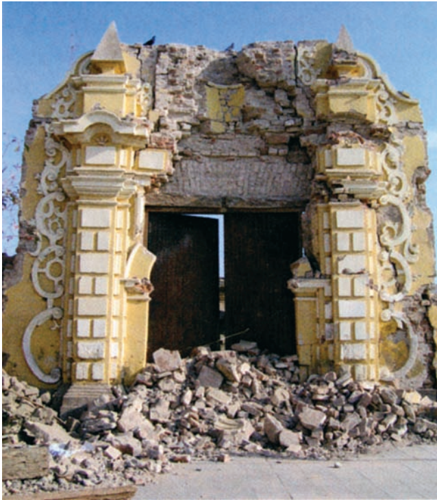
The ruined Church of the Company in Pisco (Photo: Rommel Angeles Falcon)
