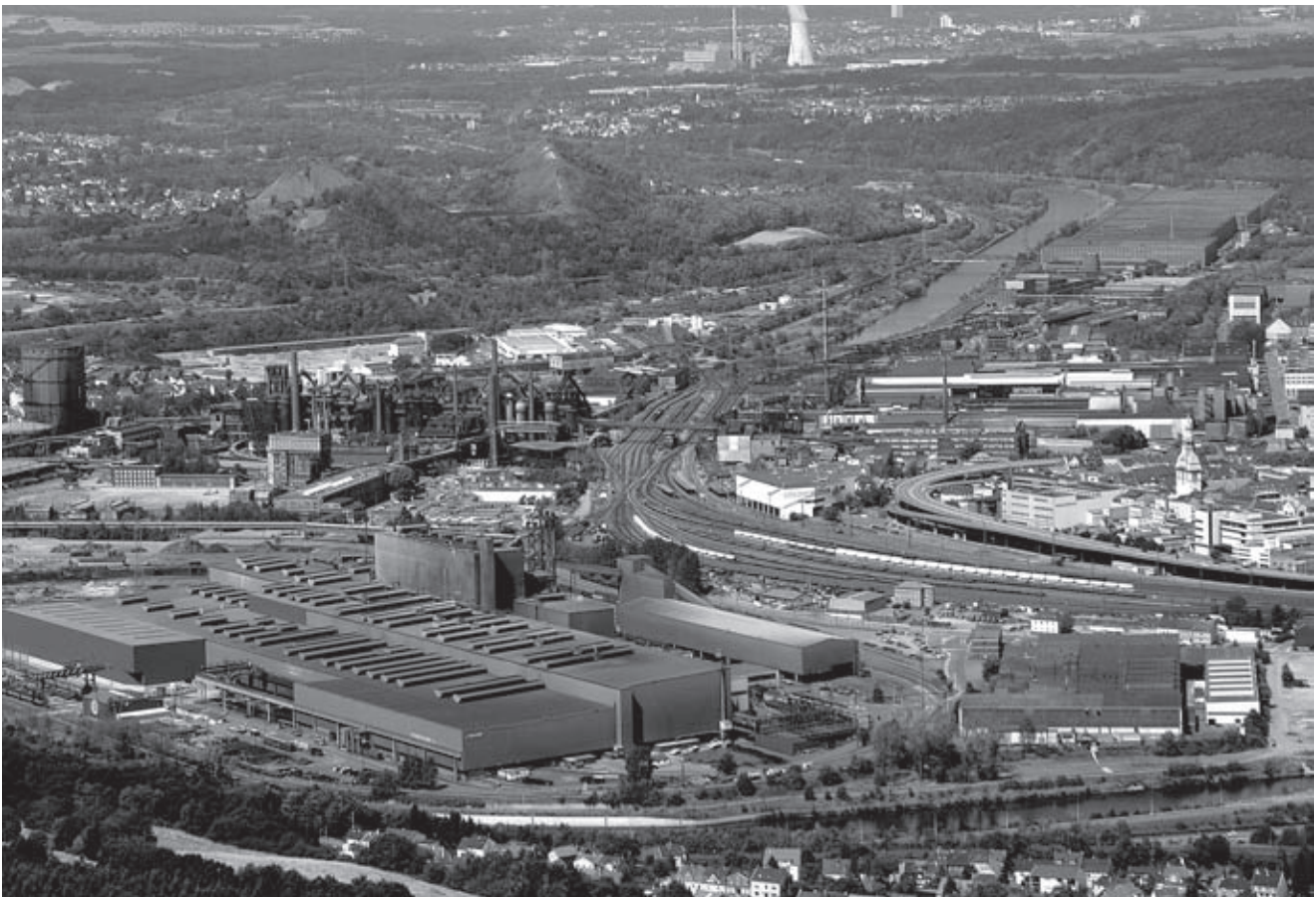
The World Heritage site seen as part of the industrial landscape of the Saar Valley, together with “Saarstahl AG” factory buildings; the modern steelworks are in the foreground
