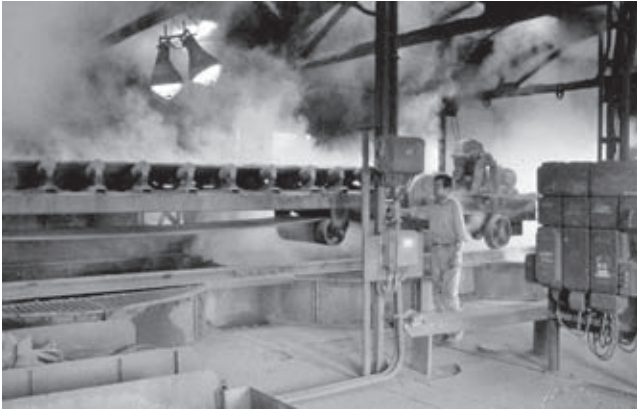
Sinter plant: the planned re-use as office space was given up in 2001 when research revealed that too many interventions into the historic substance would have been required
