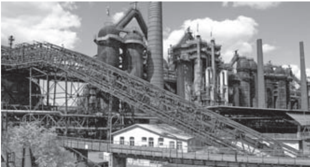
Völklingen Ironworks. Detail view
