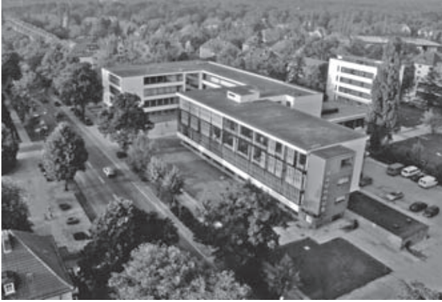
Bauhaus Building, Aerial overview, 1997
