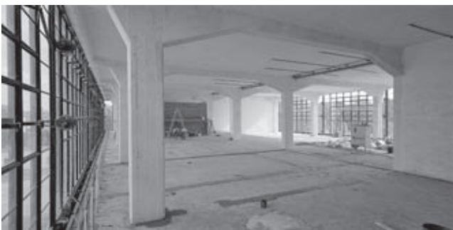
Bauhaus Building construction site, workshop wing, 2005
