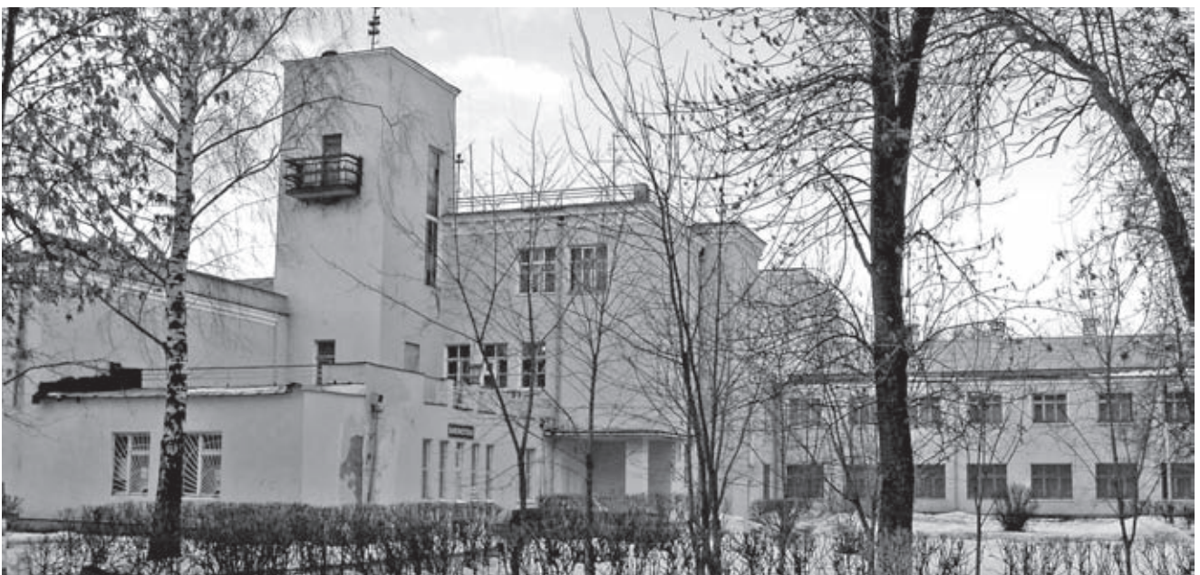
Metal workers club in Podolsk near Moscow, 1927–29, arch. I. Ivanov-Shits
