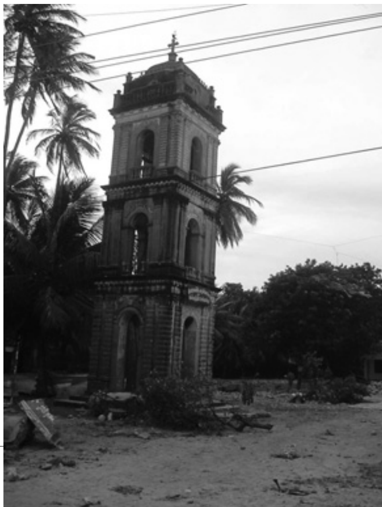
Church in pt. Pedro that has survived the tsunami
