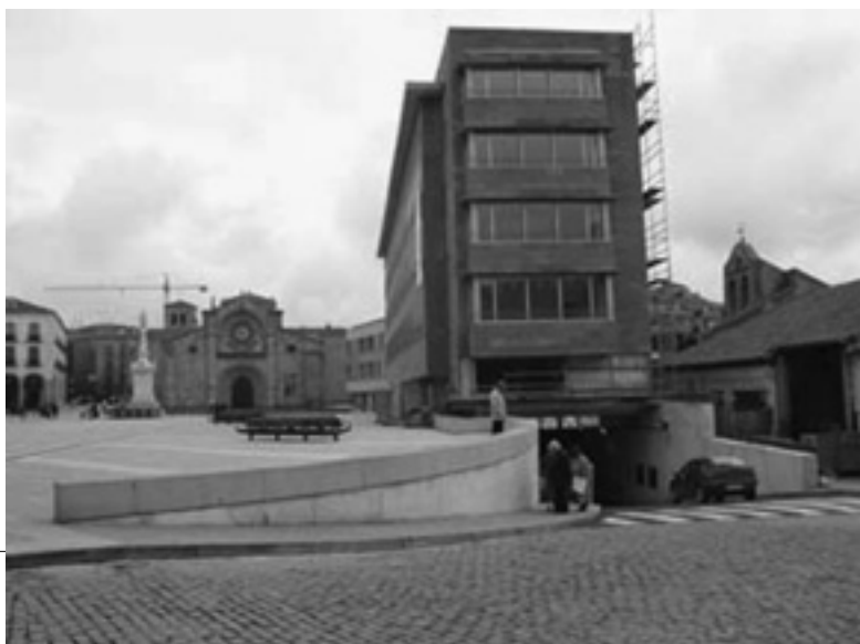
Avila, Plaza de Santa Teresa (Mercado Grande), on the right new building 'A' with entrance to the parking area
