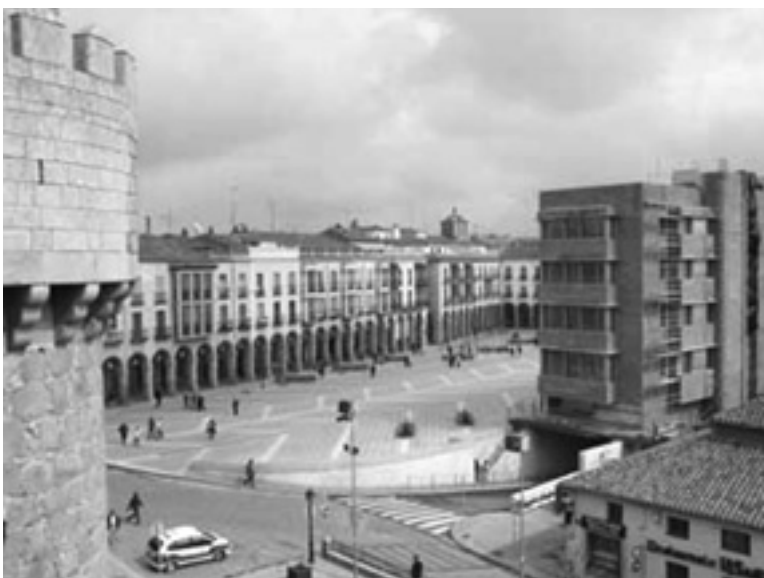
Avila, Plaza de Santa Teresa (Mercado Grande), on the right new building 'A' with entrance to the parking area
