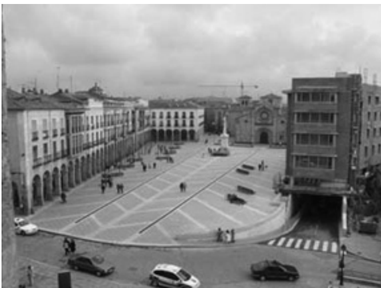
Avila, Plaza de Santa Teresa (Mercado Grande), on the right new building 'A' with entrance to the parking area
