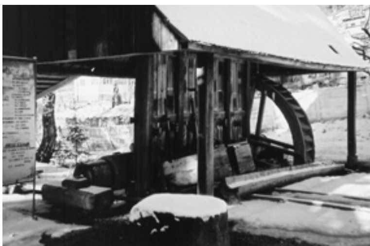
Roşia Montana, 17th-century stone breaking mill
