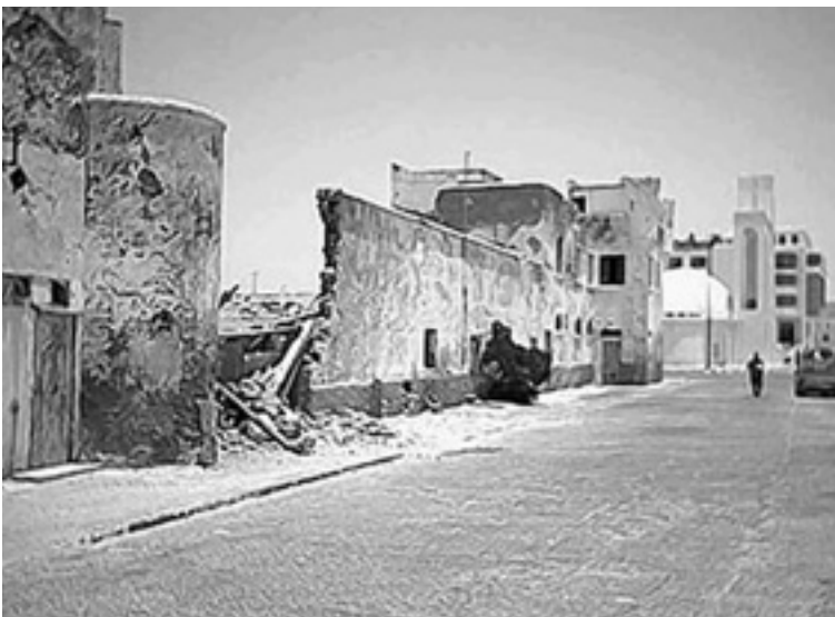
Demolition of a wall of the fort
