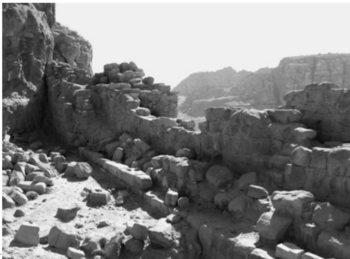
Palace Tomb: Elements, which have been masoned, not cut from the rock
