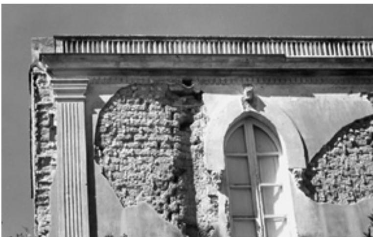
Erosion of mudbrick caused by neglect and lack of maintenance of downpipes and gutters (Samatzai, Sardinia)
