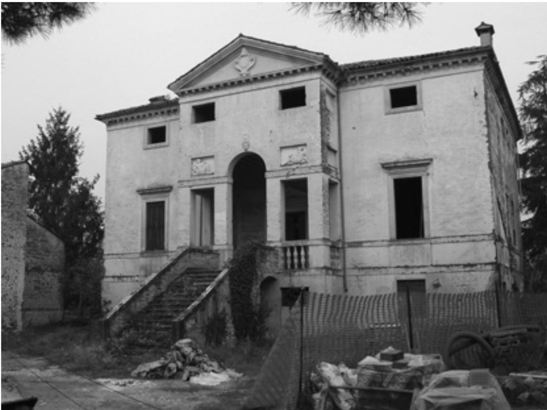
Villa Forni-Cerato in Montecchio Precalcino near Vicenza, a building by Andrea Palladio (1541-2). A piece of World Heritage in an increasing state of decay (leaking roof, no windows, the dilapidated interior with endangered wall paintings).
