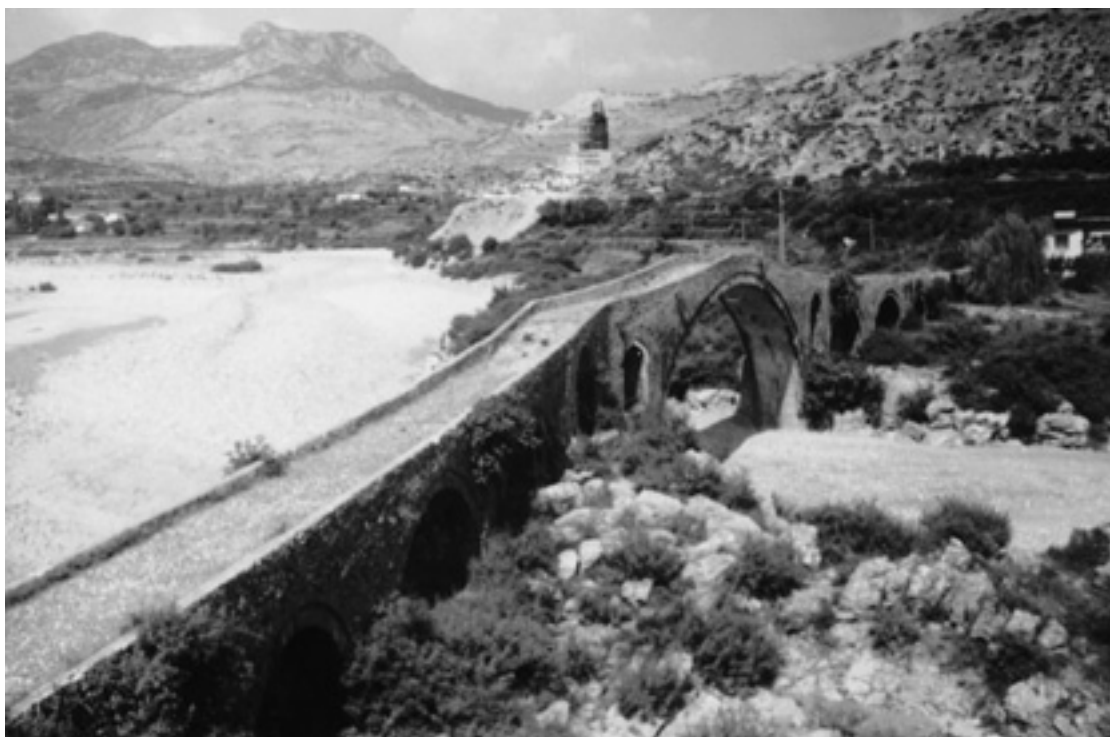
View of the Mesi Bridge at Shkodra
