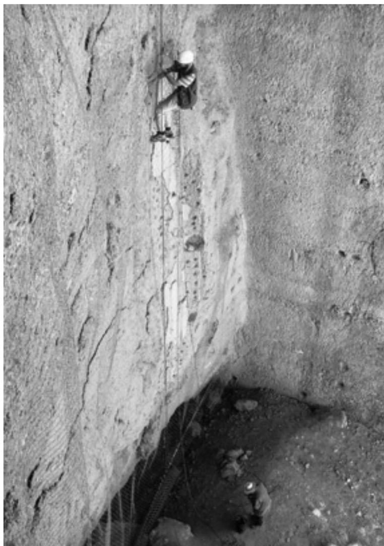
Provisional fixing of plaster fragments on the back wall of the niche of the Small Buddha, carried out by restorer E. Praxenthaler
