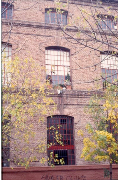
Figure 2. Lofts de Darwin, formerly the Casa Dall'Acqua textile factory (Photo: Stella Maris Casal)
