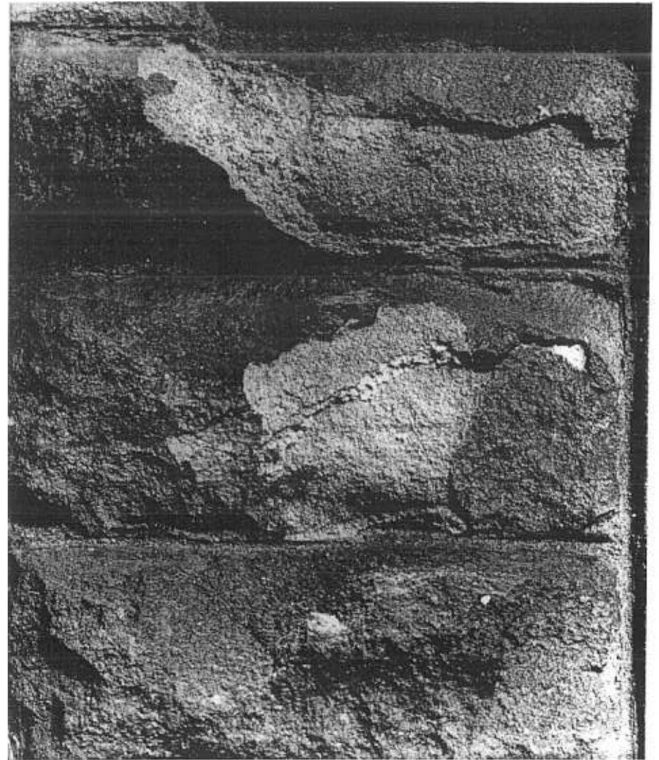
Fig. 1 - A common problem. Decaying ancaster oolitic limestone. Grantban, Lincolnshire (England).
