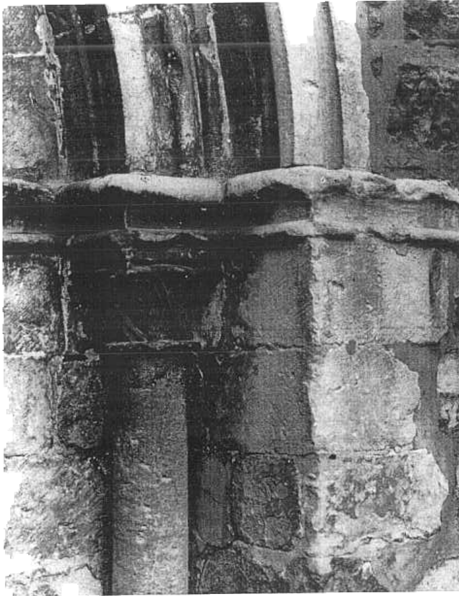
Fig. 2 A common problem. Dissolving caen oolitic limestone. Ewburst, Sussex (From France).
