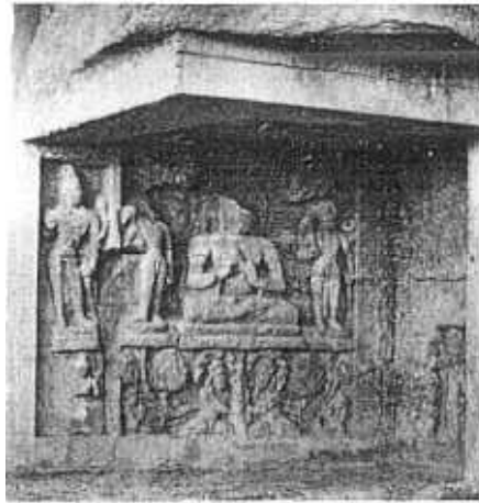
Pl. 5 - Ellora. The cell after introduction of R.C.C. beam to support the roof and removal of the pillar.
