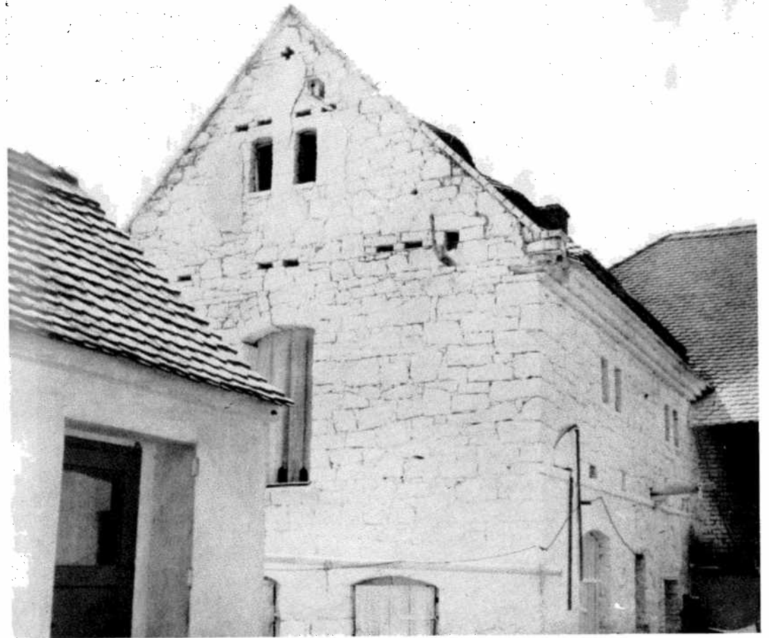
5. A storeyed stone barn made from tufa (a room for drying hops in the upper storey). Lipenec (nr. Louny)
