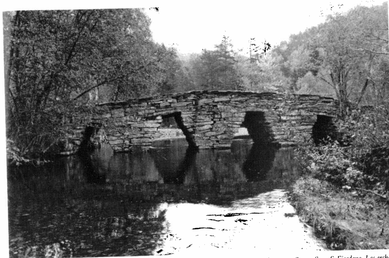
Stone bridge at Sinderøyane, Stryn, Sogn & Fjordane. The arches are constructed with projecting dry-stone corbelling. Bridges are just one of many types of technical monuments which must be added to the list of protected buildings and monuments if this is to give a more complete picture of our past. Because of their size, bridges like this are unable to take modern vehicles, but light traffic and pedestrians present no problem. Once they have been repaired and consolidated, they require a minimum of maintenance and can continue to tell their story for a very long time to come, as well as being a sculptural attraction in the cultural landscape.
