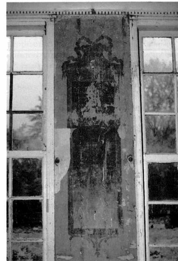
Beneath later layers of paint an imitation Louis XVI mirror in «mahogany» and «intarsia» had been painted on the original 1797 surface between the windows.
