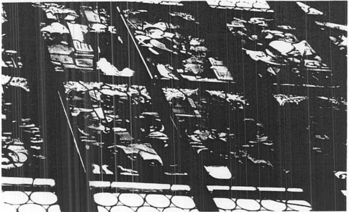
6. Nürnberg, St. Lorenz, süd XVI; isothermal glazing as a most effective protective method to ensure conservation.
