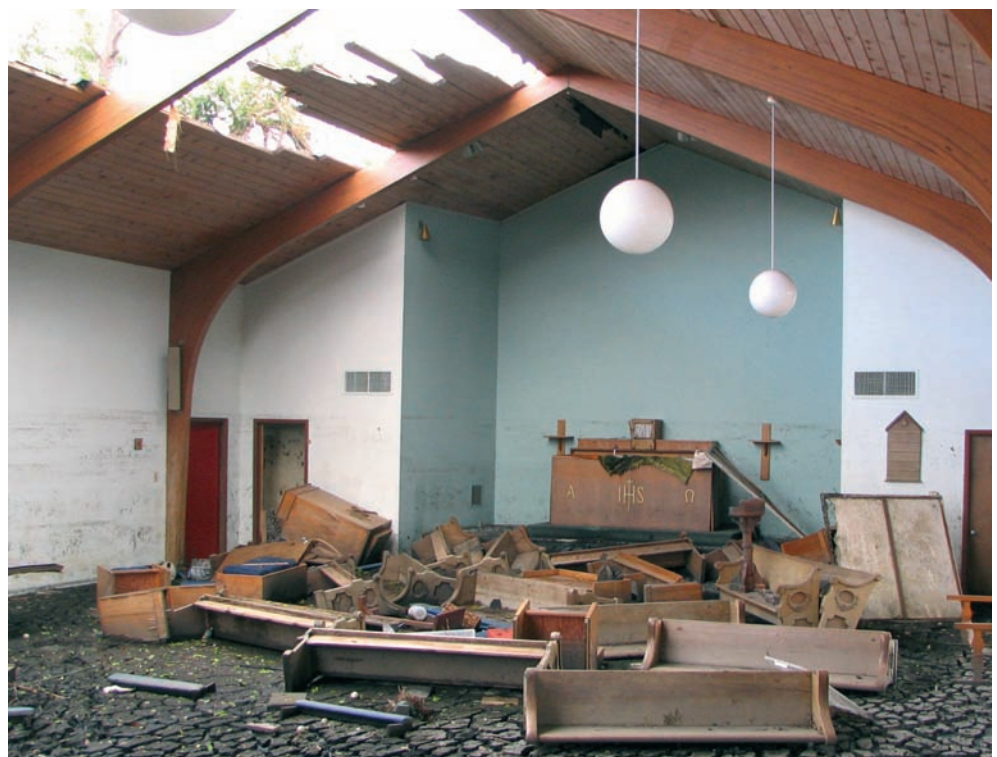
Fig. 5 Image inside of a church in the Ninth Ward after the flood had subsided. Wind damage can be seen on the roof and sediment from the flood has "raised" the level of the ground by about 3 cm.
