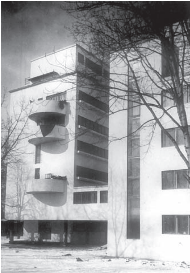
Narkomfin commune house of the Ministry of Finance on Novinsky Boulevard 25, Moscow, arch. M. Ginzburg, I. Milinis, 1928–30. View from South, 1930
