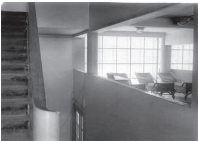
Narkomfin commune house of the Ministry of Finance on Novinsky Boulevard 25, Moscow, arch. M. Ginzburg, I. Milinis, 1928–30. Interior of the communal block. 1930
