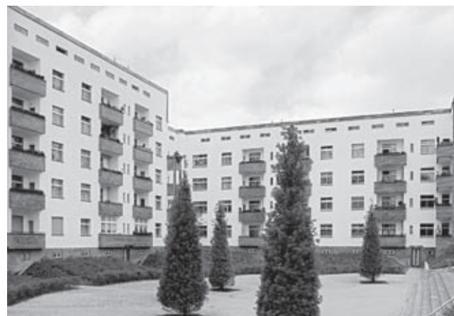
Housing block Ernst-Fürstenberg-Strasse, courtyard, after restoration, 1998
