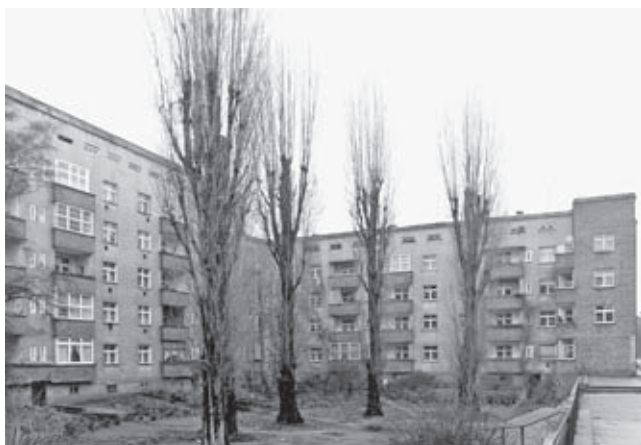
Housing block Ernst-Fürstenberg-Strasse, courtyard, before restoration, 1997
