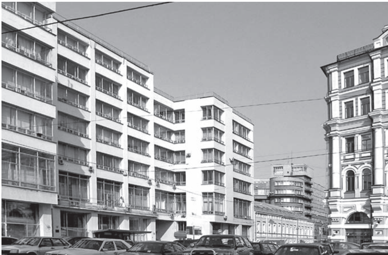
Gostorg Ministry of Trade, Mjasnitskaya street 47, Moscow, arch. B. M. Velikovskiy, A. J. Langman, M. Barsch, 1925–27, monument of local importance. Narkomsem Ministry of agriculture, arch. A. W. Schusev with Bulgakov, Franzus, Jakovlev, 1929–33, monument of local importance, in 2005
