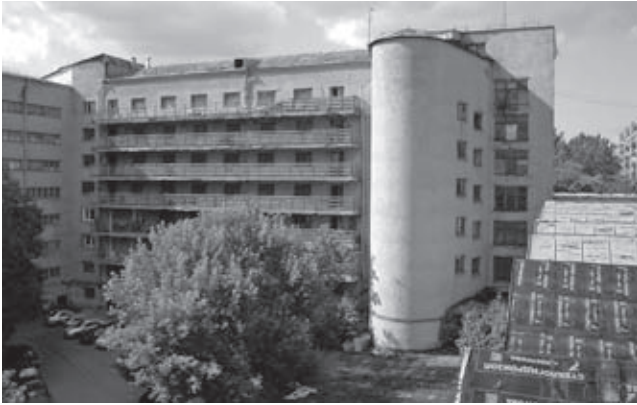
Commune house for textile institute students on Ordzhonikidze street 8–9, Moscow, arch. I. S. Nikolaev, 1929–30, monument of local importance. View from the roof of the institute in 2005
