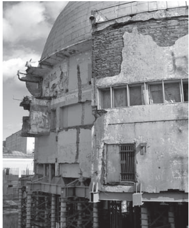
Planetary, Sadovaja-Kudrinskaya Street 5, Moscow, arch. M. O. Barsch, M. I. Sinjavsky, 1927–29, monument of local importance. In 2004 the cupola was hydraulically raised six metres to create more space. The original annexes were removed and re-constructed
