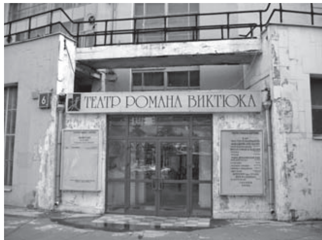
Rusakov workers club, Stromynka Street 6, Moscow, arch. K. Melnikov, 1927–29, monument of local importance. Main entrance with plastic doors, 2005
