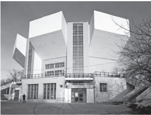
Rusakov Workers' Club in Moscow, arch. K. Melnikov, 1927–29. Condition in 2005
