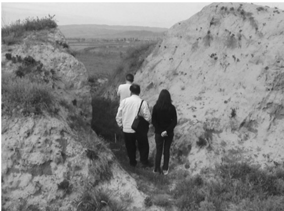
A part of the pradakshina patha with the highly threatened mudbrick structures of the cella (left) and the outer wall
