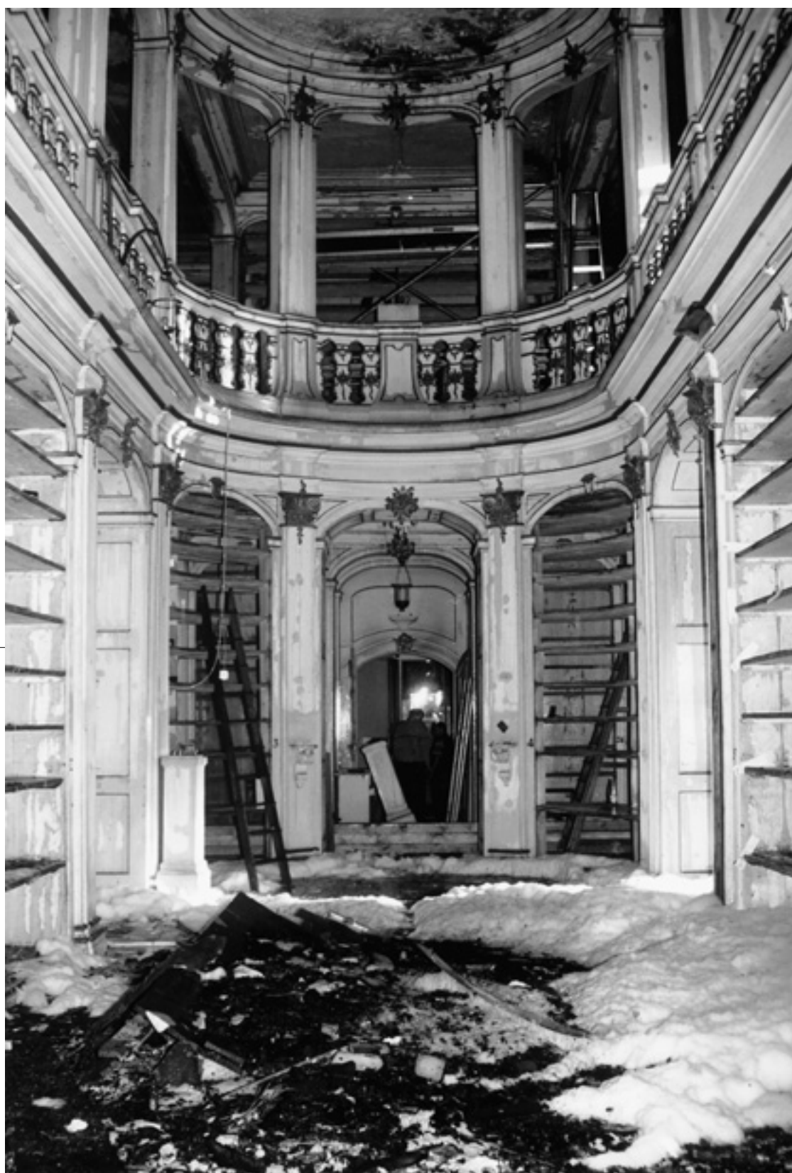
The cleared-out Rococo hall after the fire with remains of debris and foam as well as with provisional shoring (photo: J. Seifert)
