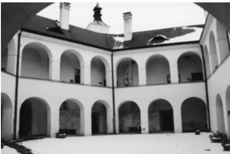
Roztoky, the manor house, the main building courtyard
