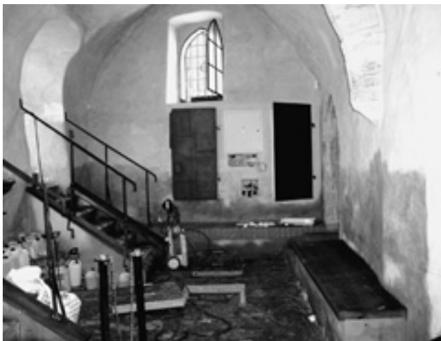
The southern hallway is the oldest addition to the Synagogue, it originated, evidently, already during the construction in the last quarter of the 13 th century. The condition shortly after the falling off of water during the 2002 flood.
