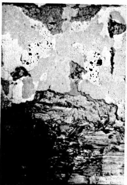
Fig. 8. It was very usual to plaster the walls inside especially in sleeping rooms to make them warmer. The plaster was generally made of earth mixed with straw like in this picture. Chaff, shives and manure were also used, and saw dust. The plaster was painted with distemper.
