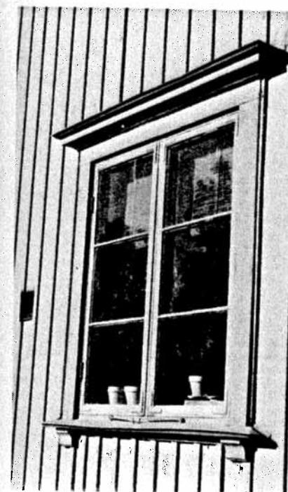
Fig. 7. Original windows were often built flush with the facade.
