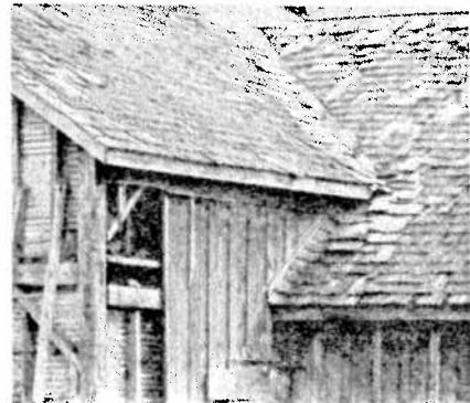
Fig. 14. Vertical board and batten mid 19th century. Ontario *en charpente* or half-timber frame. Scandinavian origin.
