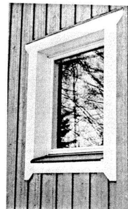
Fig. 8. After the addition of thermal insulation, new windows are recessed.
