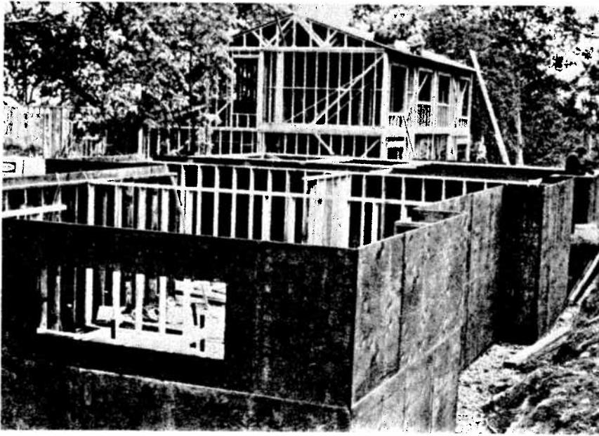
Fig. 15. The Preserved Wood Foundation (PWP) system is now rapidly gaining in popularity. The foundation is constructed for CCA or ACA pressure treated lumber and plywood.
