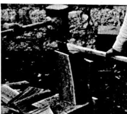
Fig. 26. Using a slitting axe or froe to split riven boards.
