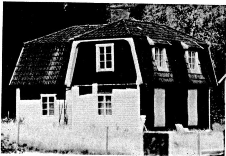
Fig. 3. Falum Red was the traditional exterior paint for wooden buildings in Sweden. The addition of new light coloured thermal insulation panels and new windows destroys the historical and aesthetic value of the building.
