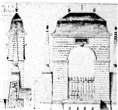
Fig. 9. Porte Frederic, 1742, Louisbourg. Wood constructed to resemble masonry.
