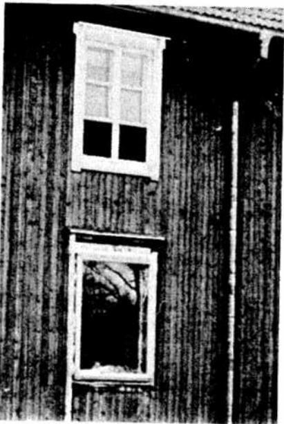
**Fig. 9.** Replacement windows often change the character of a building. The lower windows are newly triple glazed.
