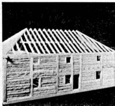
Fig. 15. Model of warehouse built of *poteaux en coulisse* also known as Red River Frame or Hudson's Bay Company Frame. Fort St. James, British Columbia.
