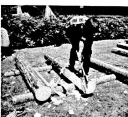
Fig. 28. Modern axe work often speeded up by a chainsaw and then finished with a broad axe.
