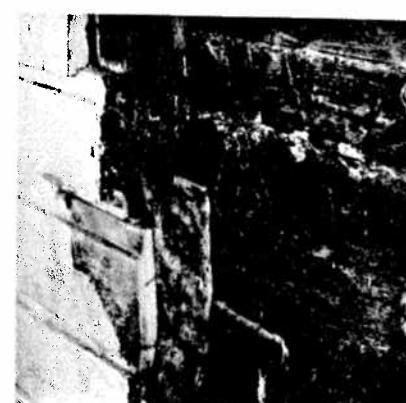
Fig. 3. A wind-proof wall from outside. The logs are well packed with oakum, with birch bark in double layers, and a tight weatherboarding overall. Degerö manor, 1818.
