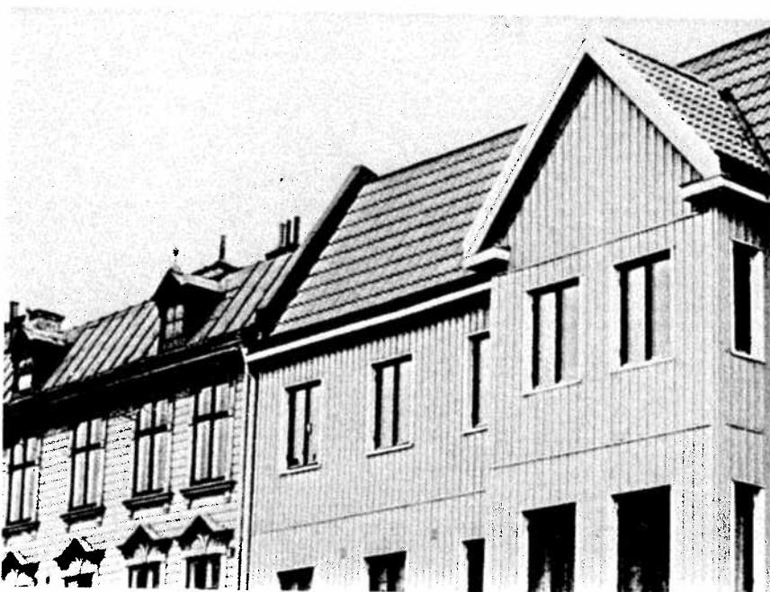
Fig. 4. New exterior insulation and new windows severely damage the building from a historical and aesthetic point of view. The two buildings in this picture originally had the same decorative elements.
