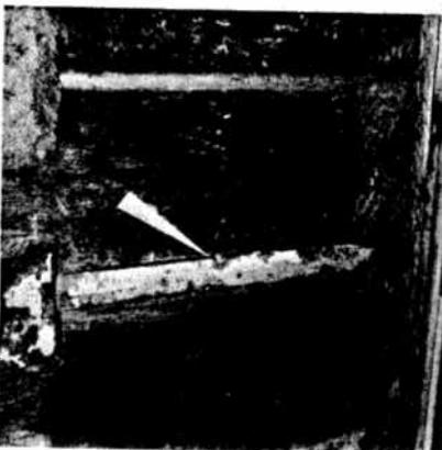
Fig. 5. The joints of logs are filled with wooden sticks. An arrow points at a wooden pin which nails the stick onto the wall. Nails made of iron were too expensive.
