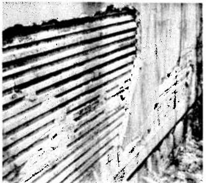
Fig. 19. Ca. 1830 southern Ontario staggered horizontal plank.
