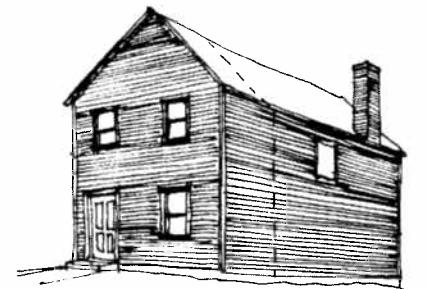
Fig. 4. A house in Halifax, N.S. which has recently been rebuilt externally, in order to remove urea formaldehyde insulation. The house was reinsulated, sheathed and clad, and extended at the same time.
