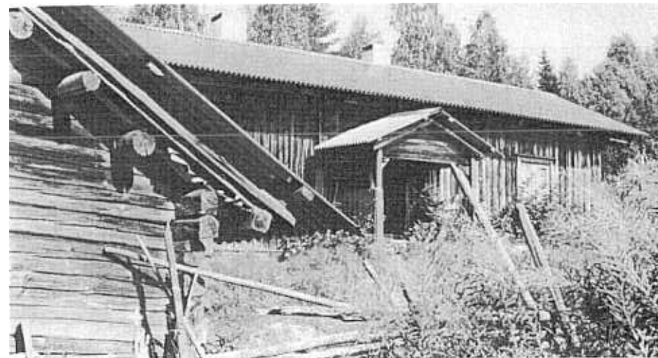
Fig. 2 The main building with its protective tin roof. The eaves might well have been longer to provide better protection against sun and rain.
