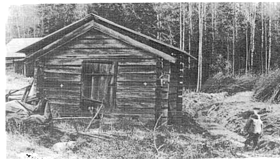
Fig. 3 This former granary (marked 1839) was standing in water every spring and autumn. Now the old ditch was opened again. The sill beams were impregnated with toxicant.
