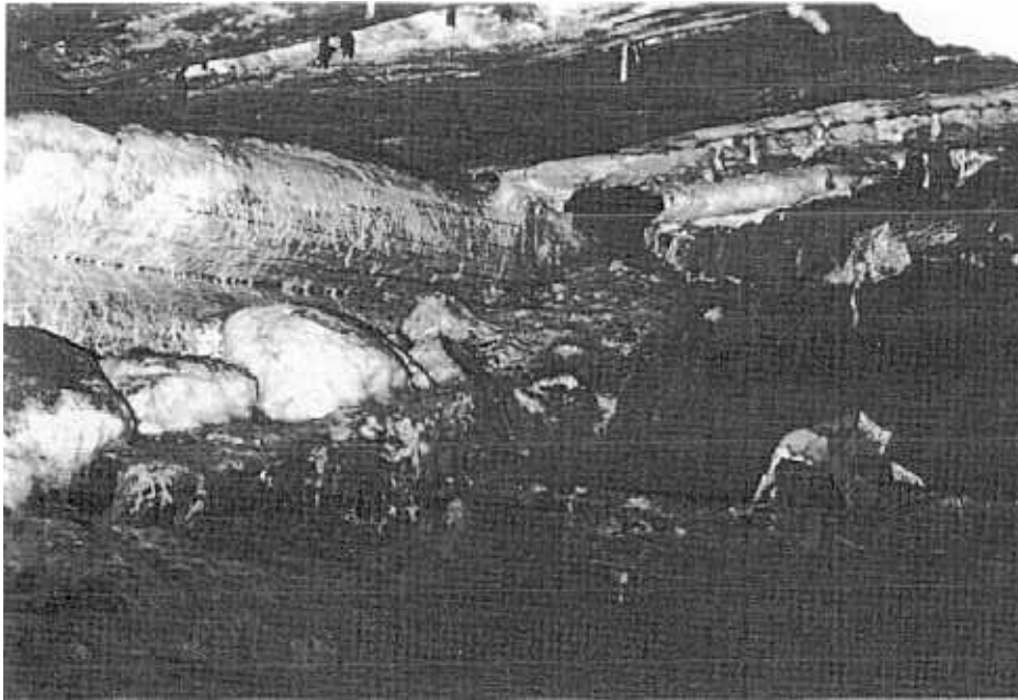
Fig. 6 The nightmare in the sub floor space. The mycelium of dry rot is covering both the wooden beams and the ground. The effort is made to eradicate it with ventilation and drainage and with some toxicants, without removing any timber.
