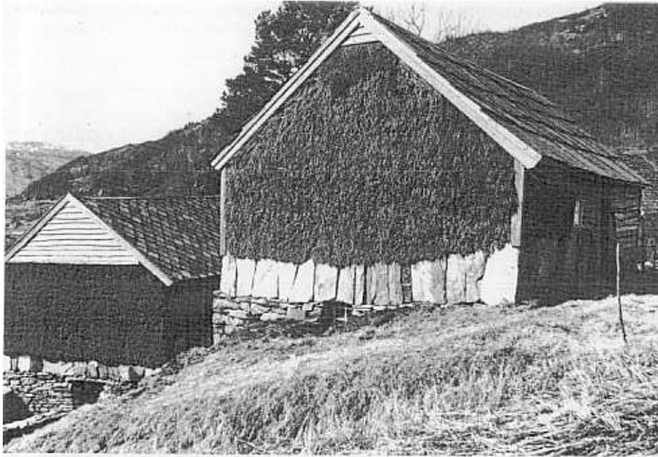
Havråtunet, Haus. Barn covered with plaited juniper twigs. Grange couverte de genévrier.
