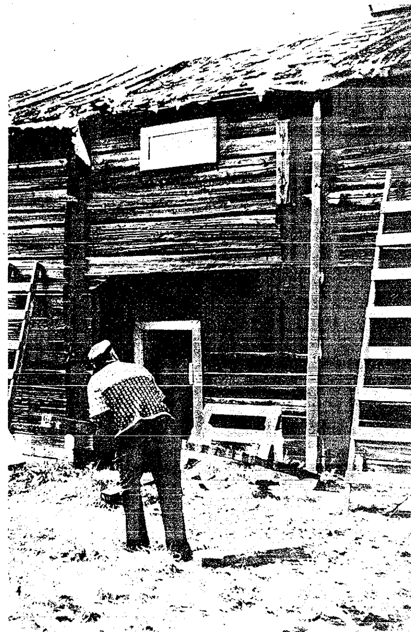
A timber house is lifted up with manpower by a simple traditional lever, so that the rotten sill beam can be replaced.
