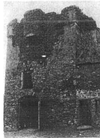
Fig. 10 - Strangford Castle, N. Ireland, before restoration.
