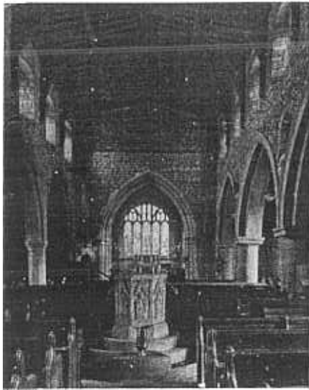
Fig. 5 - Dingy and disfiguring effect of removal mediaeval plaster.
