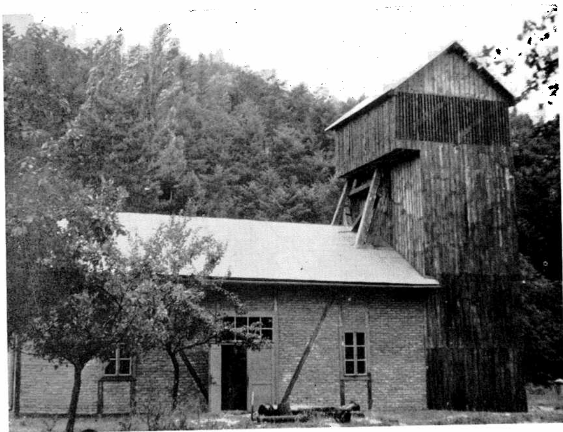
3. Mining tower with machine-room from the Mária shaft in Podsitnianská, transferred to the Open Air Mining Museum.
