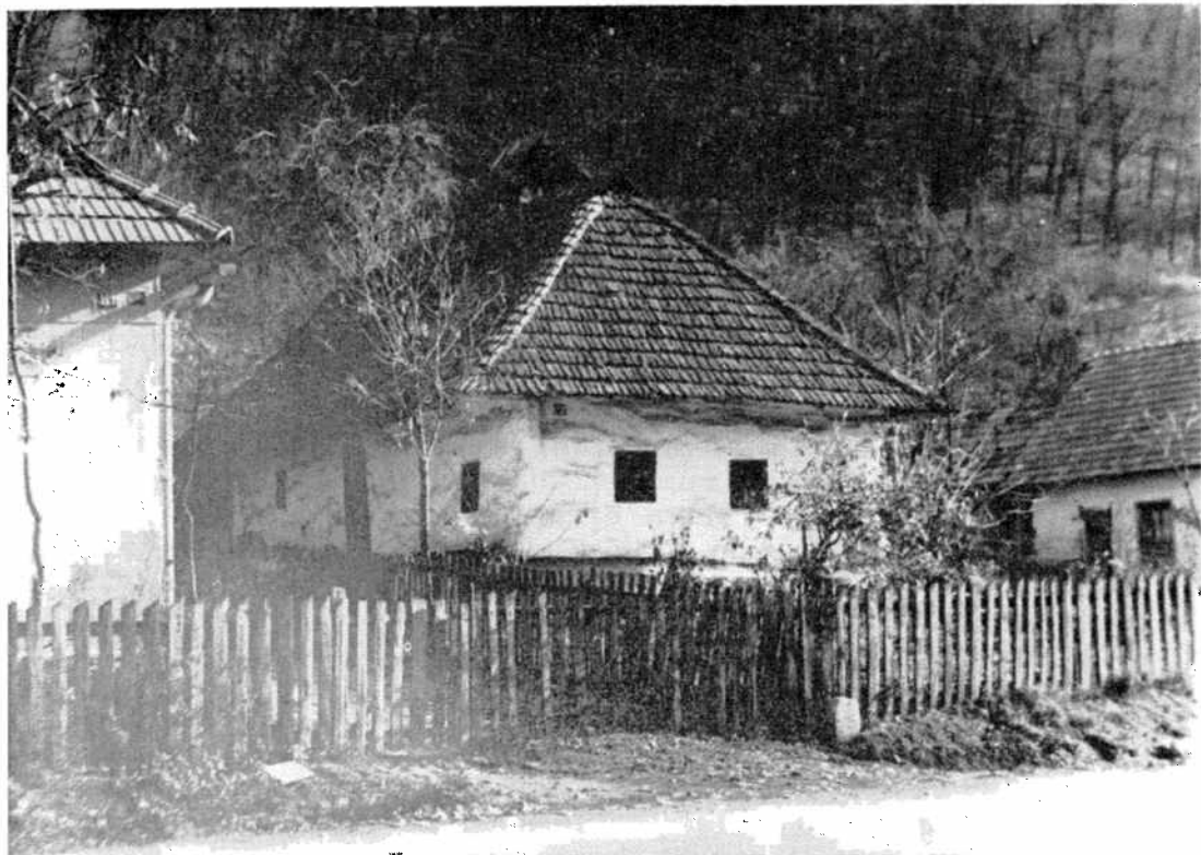
1. Miner's log cottage built from oak in the style of a Slovak house from Antol. It is about 200 years old and will be transferred to the Open Air Mining Museum.
