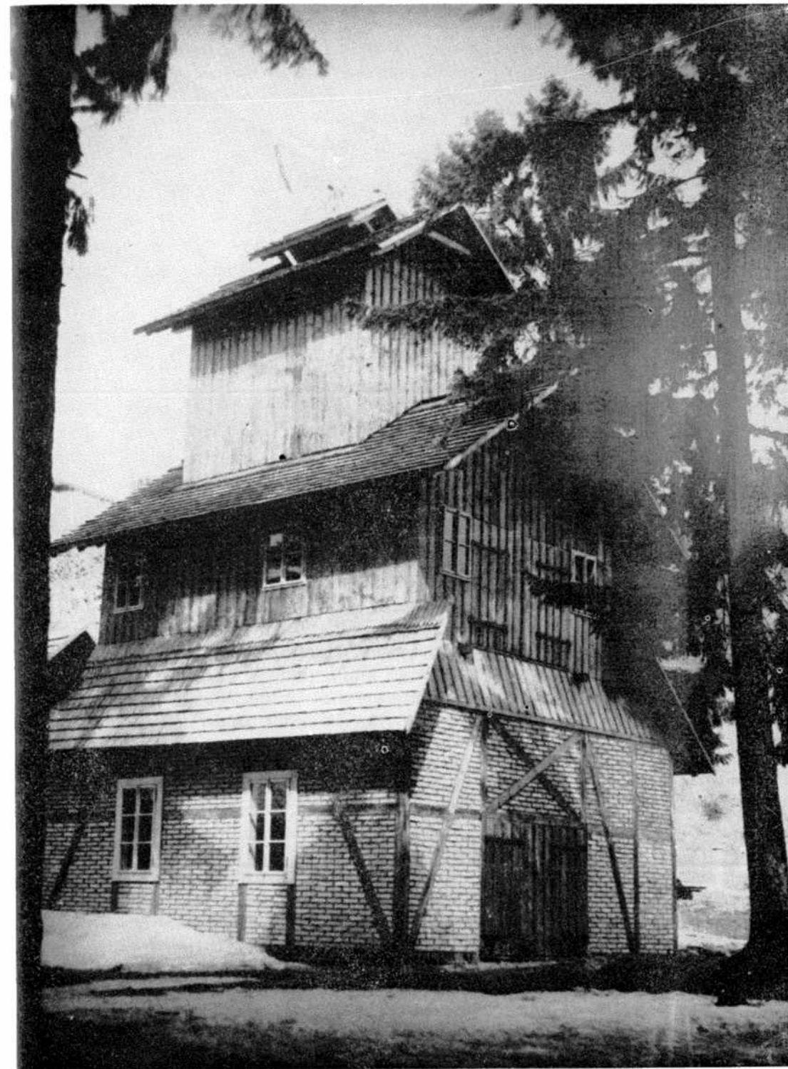
2. Mining tower from the Žofia shaft in Banská Belá transferred to the Open Air Mining Museum
