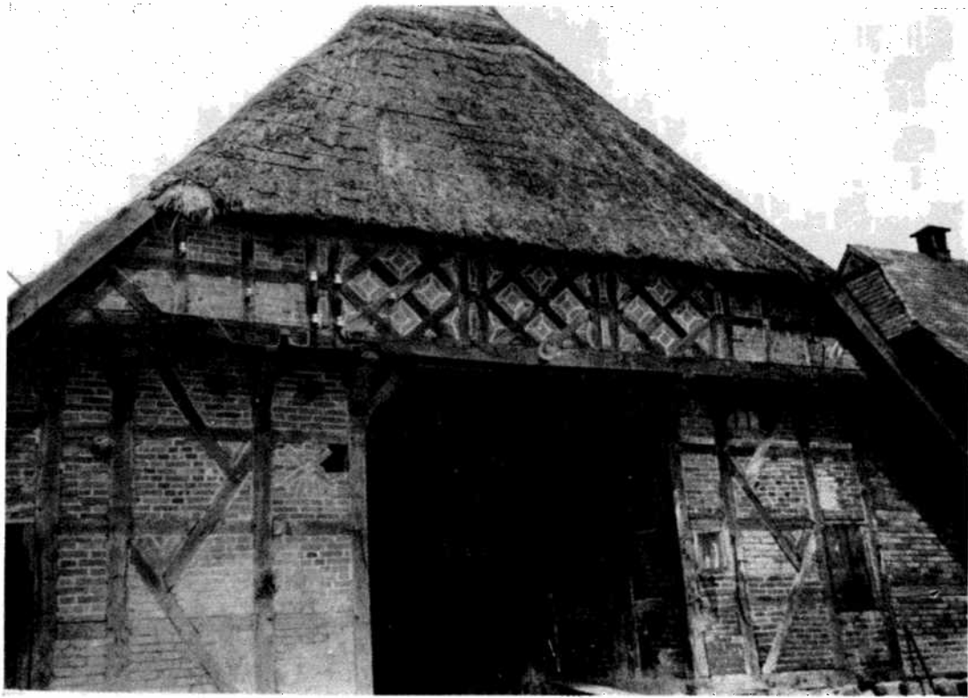
4. Thandorf, Kr. Grevesmühlen (NW-Mecklenburg) Decorative show-gable from about 1800.
