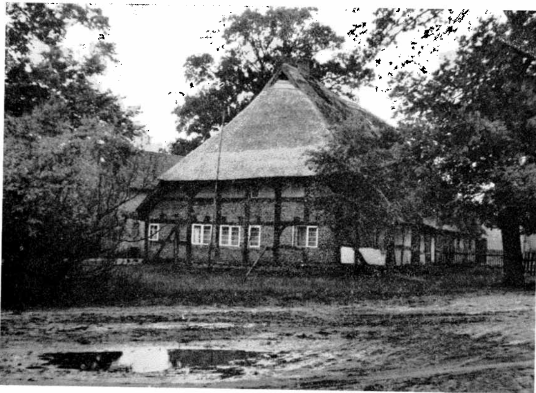
2. Stuck, Kr. Ludwigslust (SW-Mecklenburg) The rear gable with the later closed up second doorway.
