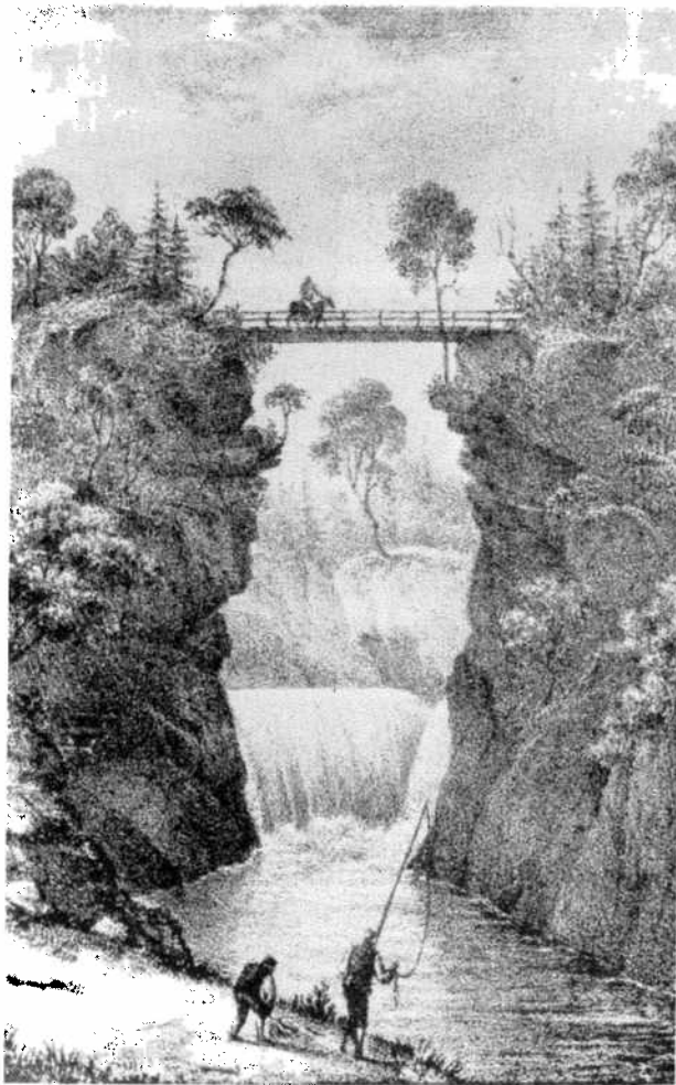
The 1951 revision of the Preservation and Protection of Antiquities Act from 1905 made it possible to protect technical installations such as roads and bridges. Tromse bridge, Fåvang, Oppland, in a lithography by Wergmann from 1855.
