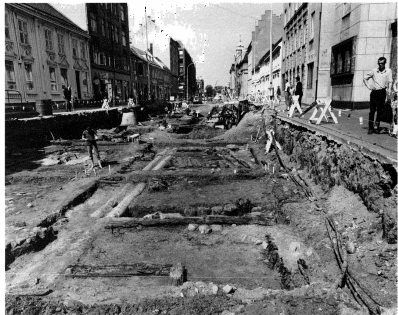
Archaeological excavation in Søndre Gate, Trondheim, 1970–71. This street was laid out in 1681 over earlier properties. Apart from the two wooden water pipes from the 1770s, down the middle of the street, all the visible woodwork belongs to pre-1681 structures.
