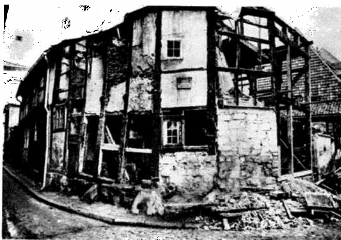
L'état de construction traditionnel – Condition before restoration
