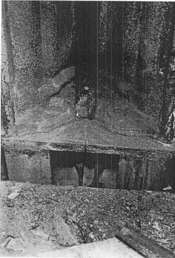
Fig. 11. — Photo of column base and bolted beams. (Photo: Courtesy H.A.B.S.)
