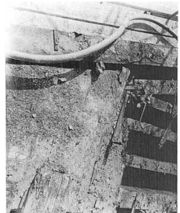
Fig. 29. — Strap irons used to secure iron front. (Photo Author.)
