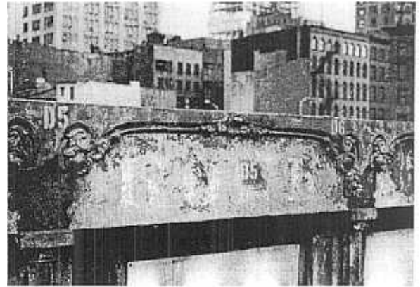
Fig. 23. — Beam ornament at 1st tier. (Photo : Author.)
