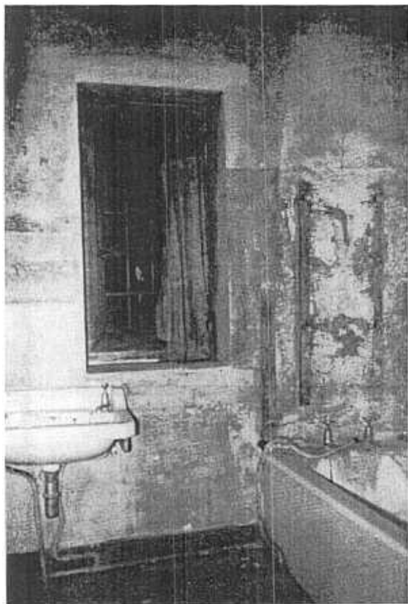
Fig. 7, 8. — The east bathroom before and after re-conditioning. The wallpaper, here and elsewhere in the Manor, is a modern
