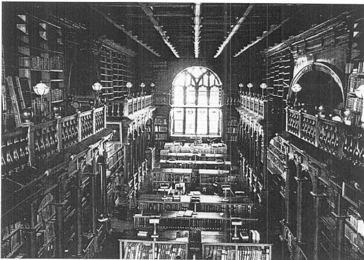
Fig. 9. — Selden End Library prior to restoration.
