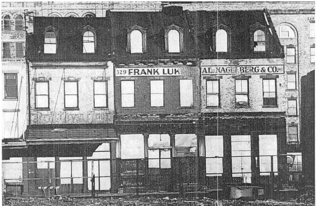
Fig. 1. — Typical urban renewal restoration problem. As a result of a hard-won campaign by New York City preservationists these houses at 327-331 Washington Street Manhattan, have been spared from the demolition that levelled the rest of the neighborhood. Substantial middle class residences of the 1820's sharing party walls, they later suffered separate remodellings with iron retail storefronts. The three houses now stand vacant and it is proposed to restore the fabrics for residential use. The student's problem was to find what the walls, doors, windows and steps looked like. (Photography by Robert E. Meadows.)
