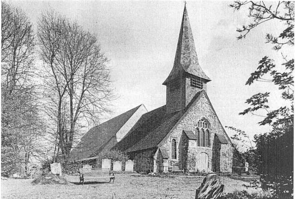
Fig. 3. — Thundersley (Essex), St. Peter. A difficult architectural problem : a 14th-century English parish church sympathetically extended by a modern nave. (Civic Trust Award, 1969).
