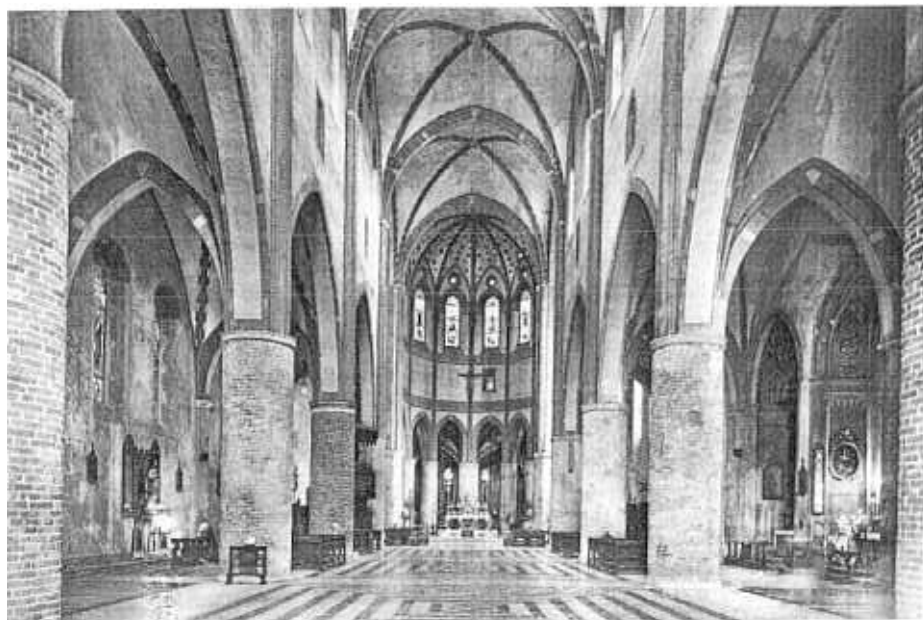
FIG. 5. Piacenza: interior of church of San Francesco (c.1278) showing the pillar in the central axis. (Photograph: Bromofoto, Milan)
