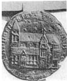
FIG. 3. Seal dating from c.1250 showing the south facade of the Martinikerk of c.1225. Actual size 6 cm in diameter.
