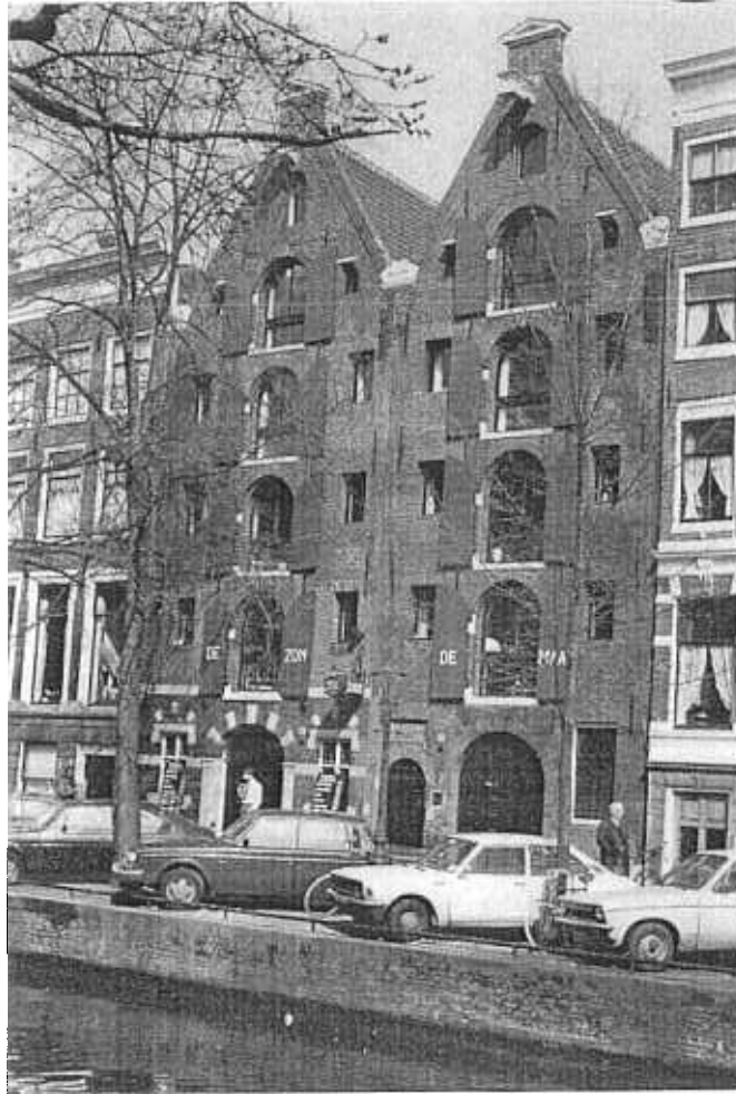
FIG. 17. 11–13 Reguliersgracht. Two typical Amsterdam warehouses restored and converted for residential accommodation and a restaurant.
