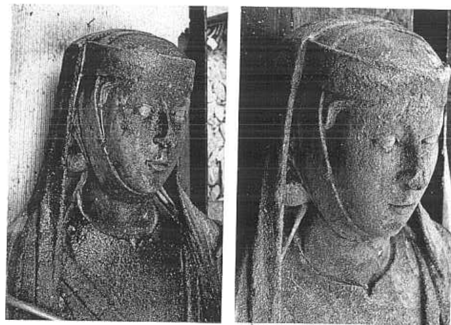
FIGS 7, 8. Before and after effect of cleaning the head of a queen at Wells with lime poultice and water. Cleaning must be followed by consolidation and protection. At this stage the detail is very vulnerable to damage.
