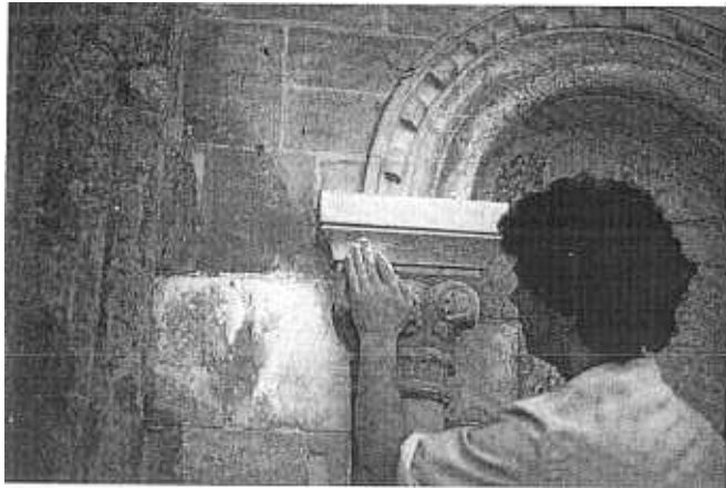
FIG. 12. Architectural detail at Christchurch Priory is shelter-coated after cleaning. The thin lime casein coat has been applied by brush and is being rubbed in by hand, using a small pad of coarse cloth.
