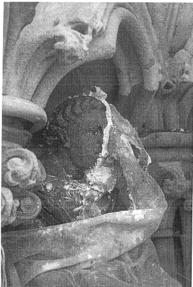
FIG. 6. The shrouds, wet bandages and lime poultice being removed from a figure at Wells. Some of the dirt detaches with the pack, and what remains will usually be more responsive than before to gentle scrubbing.
