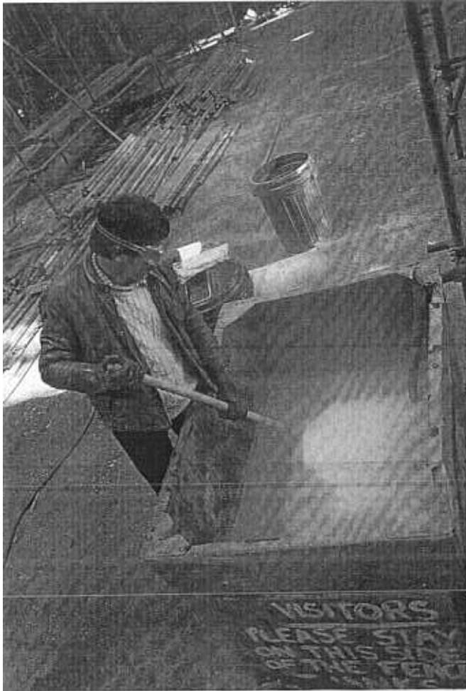
FIG. 3. The slaking tank. Lime slaked in the traditional way is the basic raw material for much of the lime method activity.
