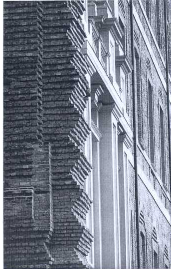
FIG. 1. Castello di Rivoli; detail of the facade showing the toothed brickwork and part of the facing of Juvarra's projected facade.
