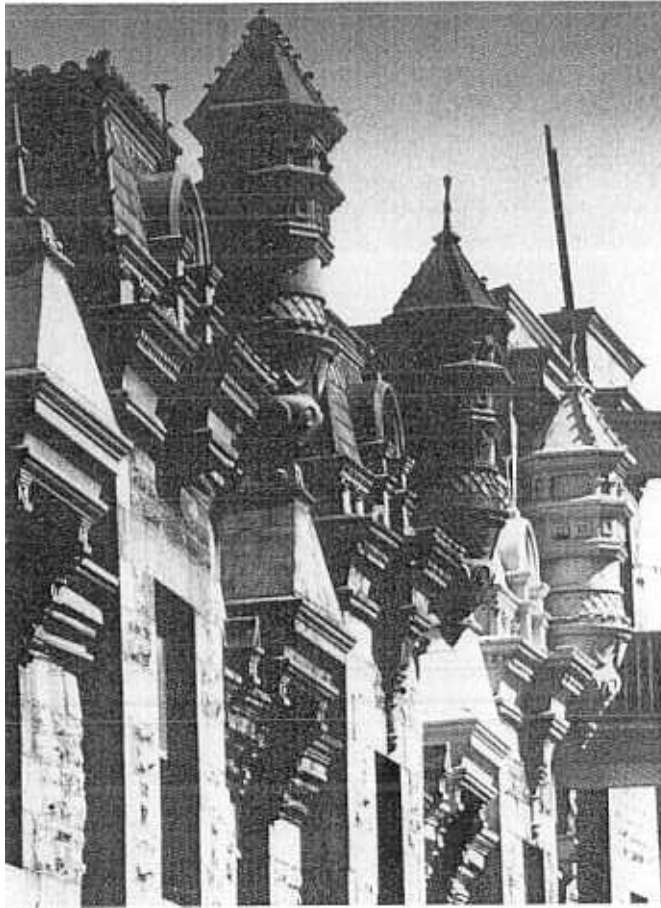
FIG. 13. A decorative roof line in Montreal.
