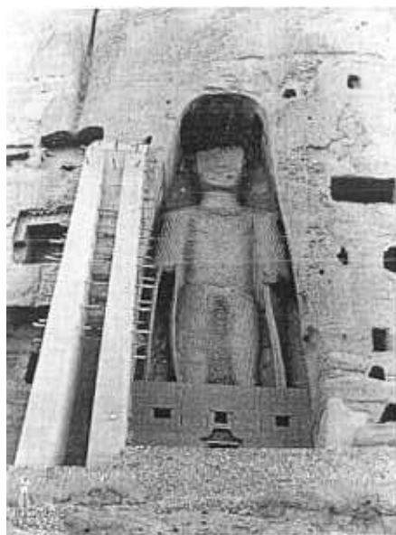
FIG. 13. The brick-faced masonry buttress wall and the modern house in front of the image.
