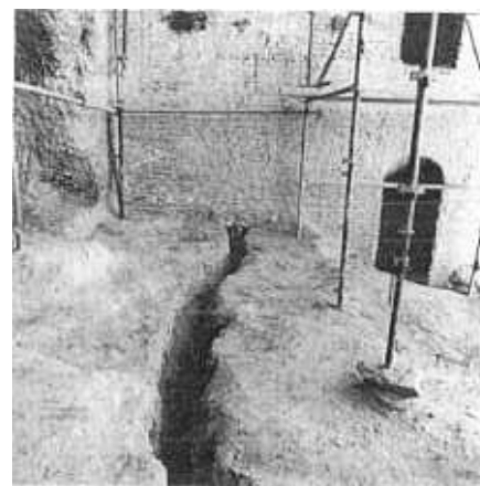
FIG. 4. A crack passing through the porch of a shrine.
